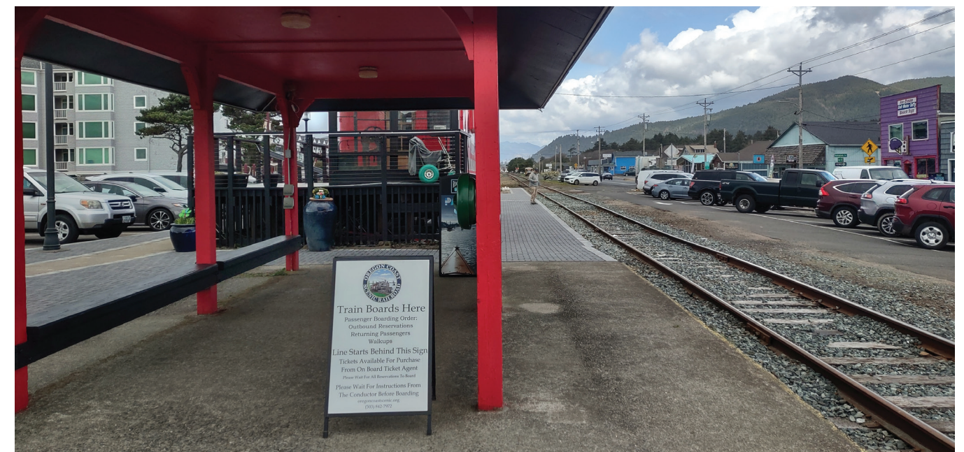
Figure 19 - Existing train boarding shelter for the Oregon Coast Scenic Rail.
