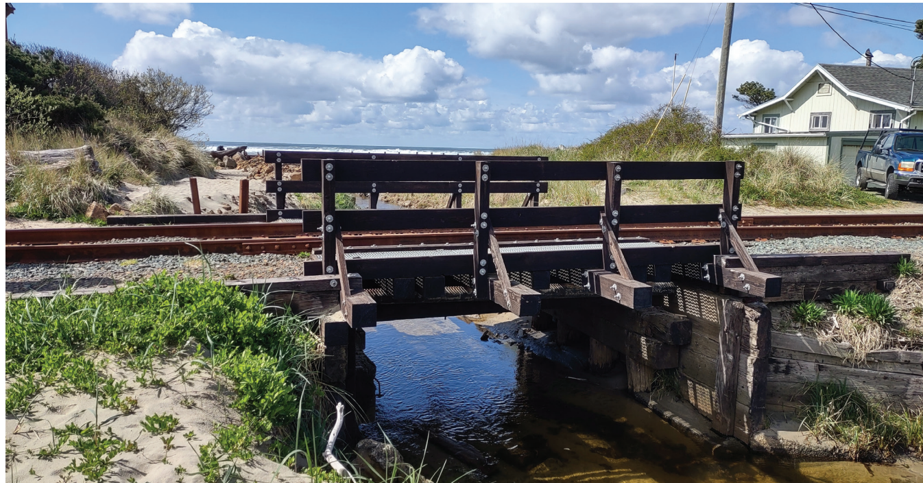
Figure 15 - Existing rail bridge over creek at the northern end of the Wayside. A pedestrian bridge is required in this location.
